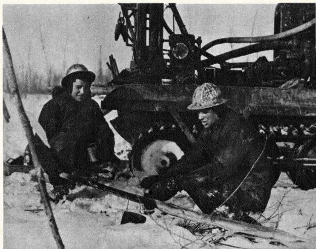
Here, two oil drillers build a fire not only to warm themselves, but to heat their tools before using them.
